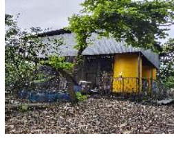
Visit to 2 TPD Biogas plant – IITB
