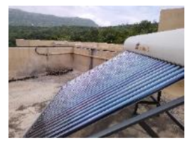
Expansion of existing Solar Heater infrastructure
